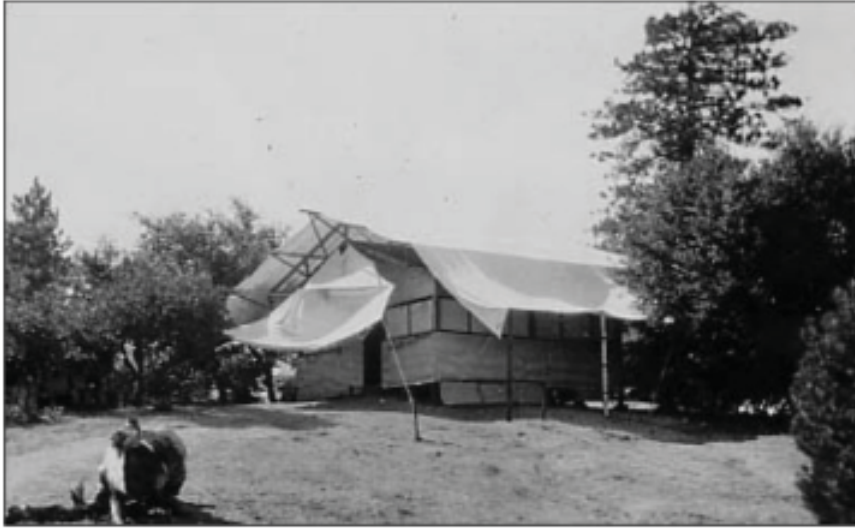
Figure 9. Miller's interferometer house on Mt. Wilson. With canvas-covered windows all around, insulating "beaver-board" walls (wood fiber composite), and fitted with a tent cover to further stabilize temperatures.
